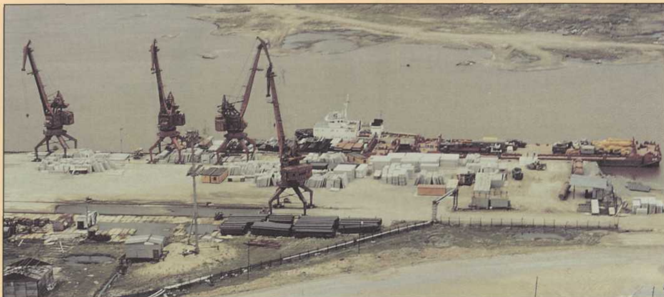
Picture: Unloading facilities at Yamburg port, Russia
