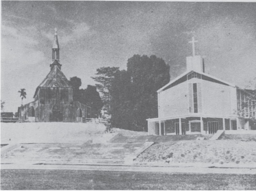
This is the cathedral of St. Thomas, Kuching which structure was built with reinforced concrete on an outer and an inner walls. The building is approximately 62 feet wide by 200 feet long. The Cathedral commands an elevated position above Rock Road, this is undoubtedly the best site possible, and it is a part of the property which was given to the church by the first Rajah of Sarawak.
