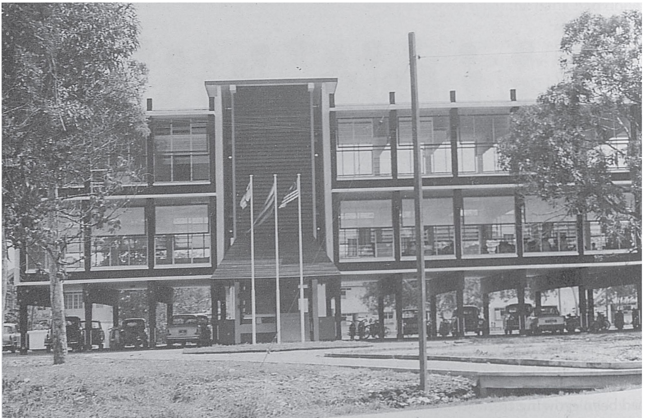
Sarawak Co-operatives Central Bank situated at Ban Hock Road, Kuching.
