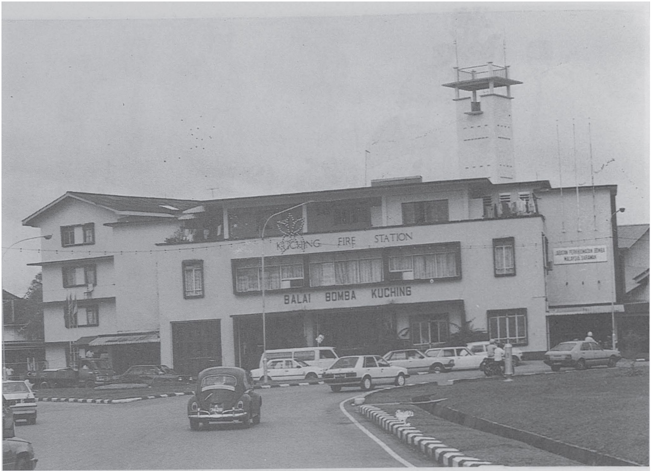
The new K.M.C. three-storey Fire Station at the junction of Central Road East and Padungan Road.
