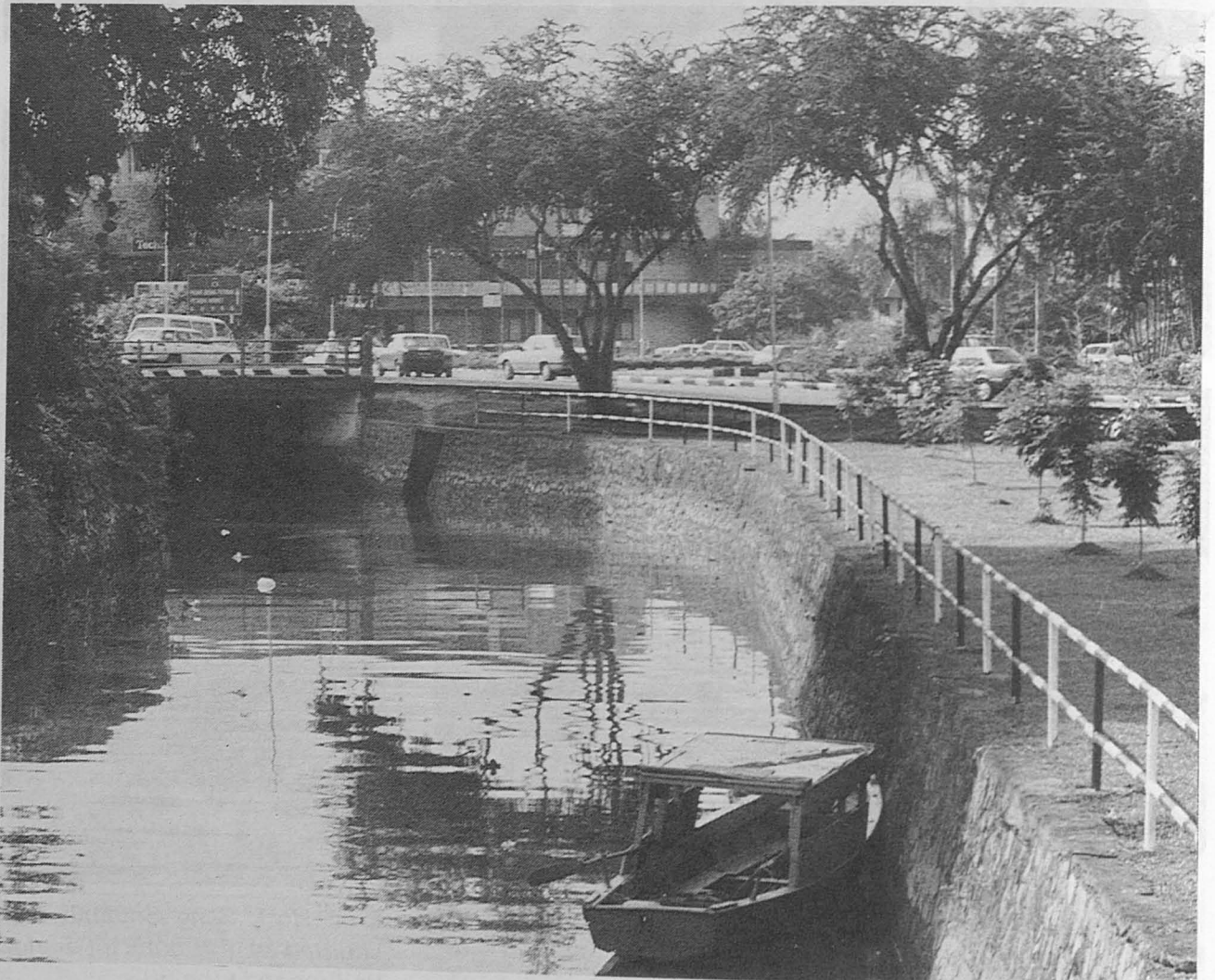
The bank of the Petanak River as from its river mouth up to the road side of Padungan Road were paved into a canal and a changed in the physical environment appeared inevitable.
