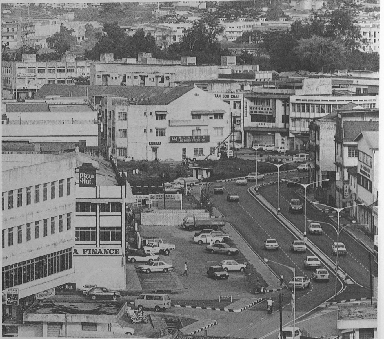
Top: The shop building at end of the Padungan road, the Kuching Fire Station, the Kuching Chung Hwa School No. 3, the Jubilee Recreation Ground, the venue for sport & football, Kuching Turf Club as a distance view.
