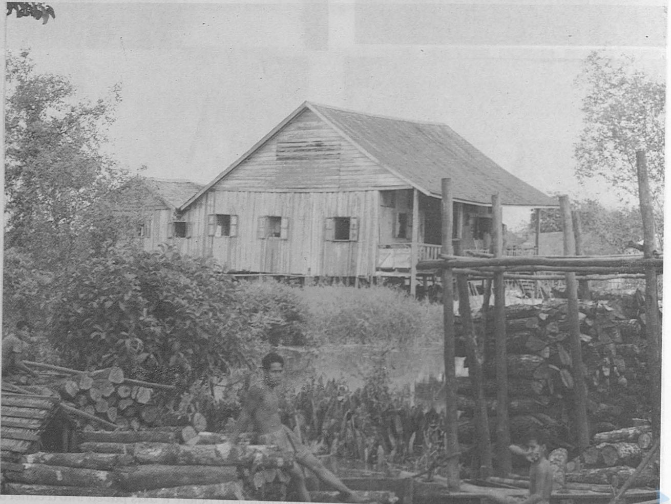
Another scene of an old wooden building along the Petanak Stream.
