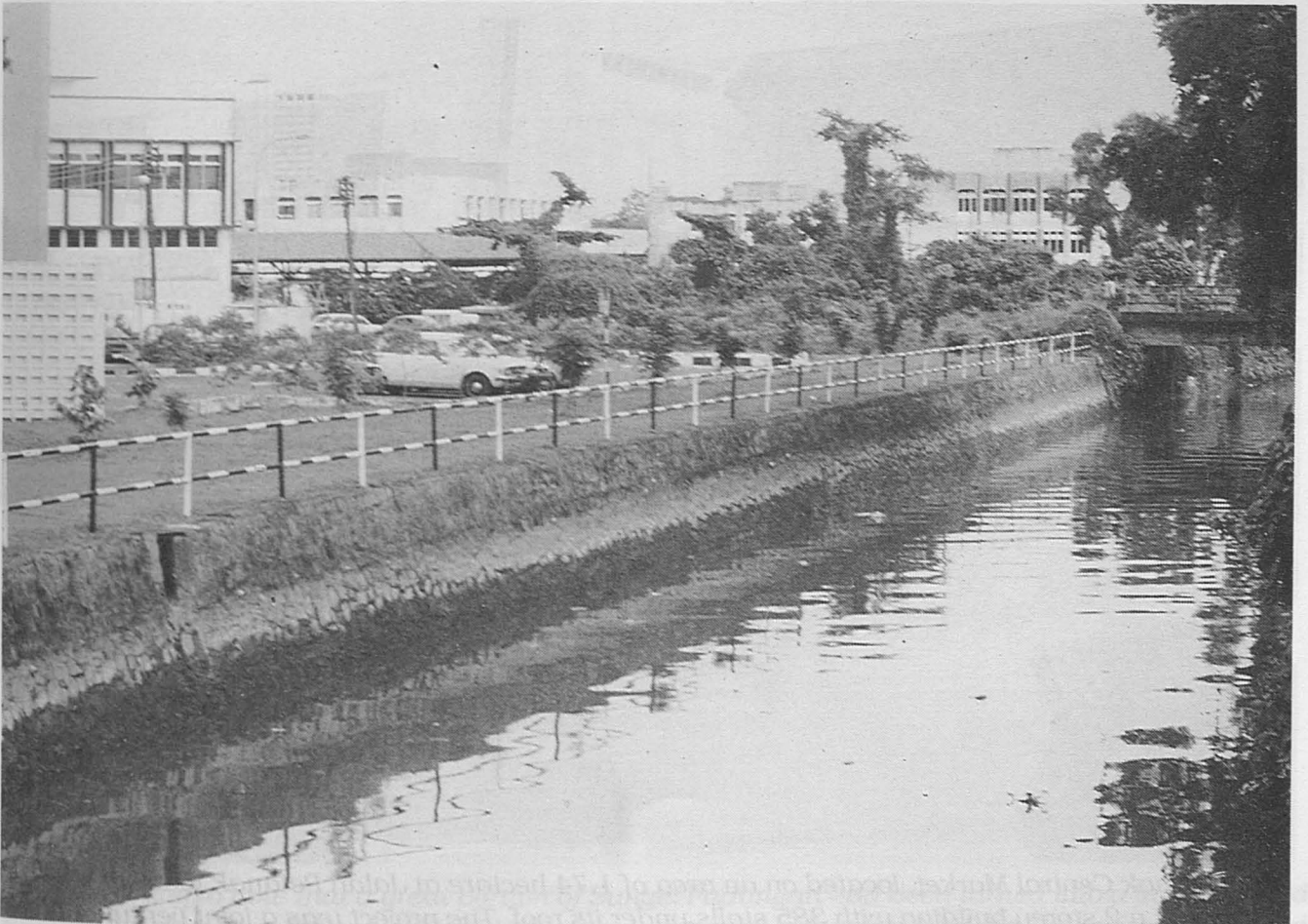
The Padungan River nicely paved like a channel.
