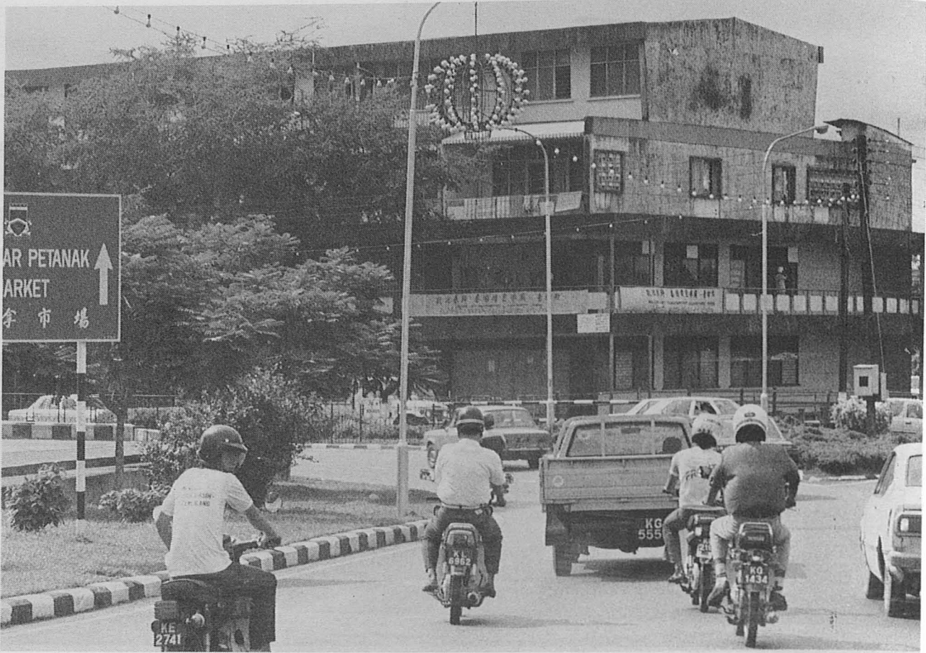
A row of new shophouses fully occupied the former Roman Catholic Mission's swampy land and building therein.
