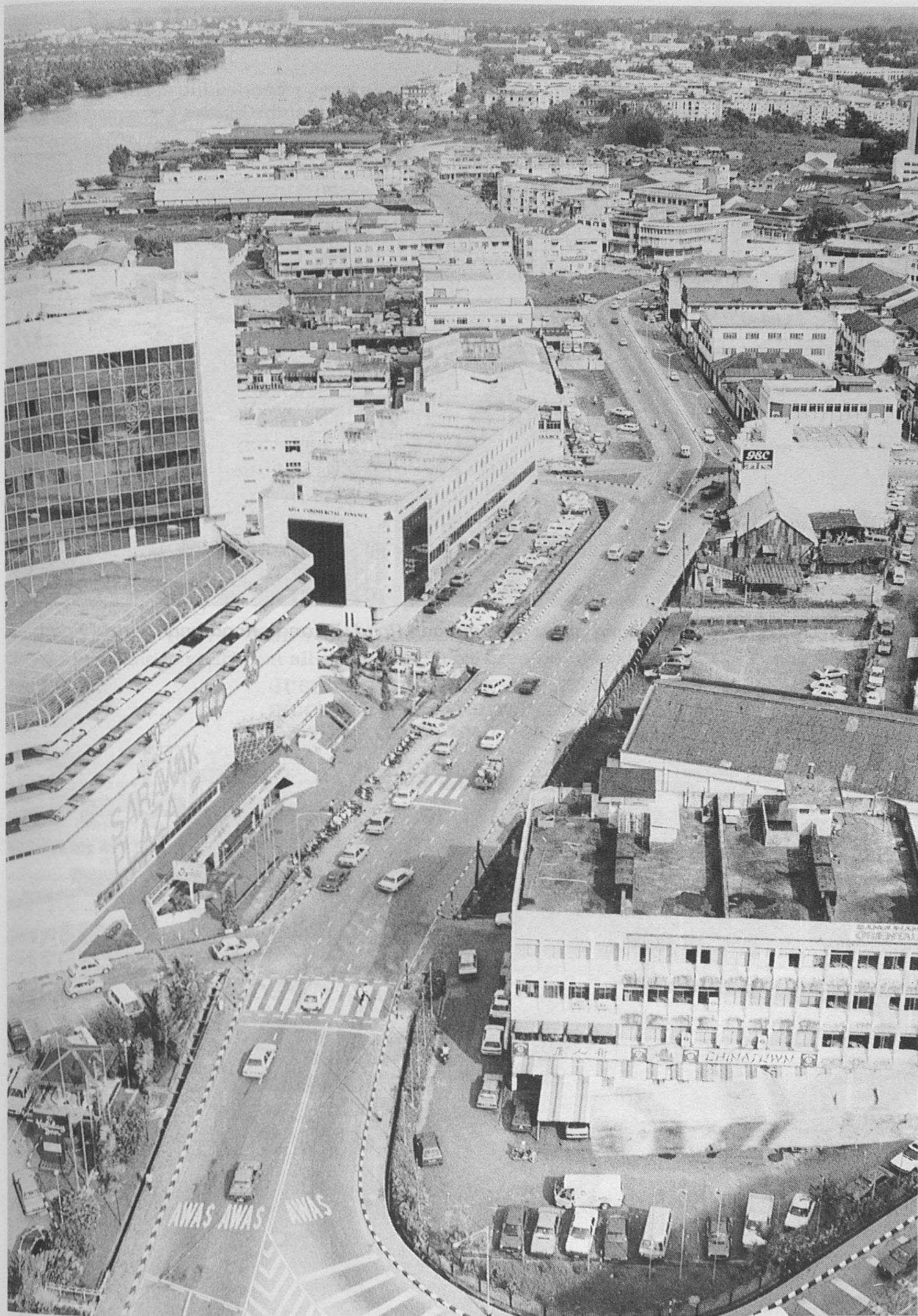
Bird's eye view of a section of Padungan building along Sarawak River.
