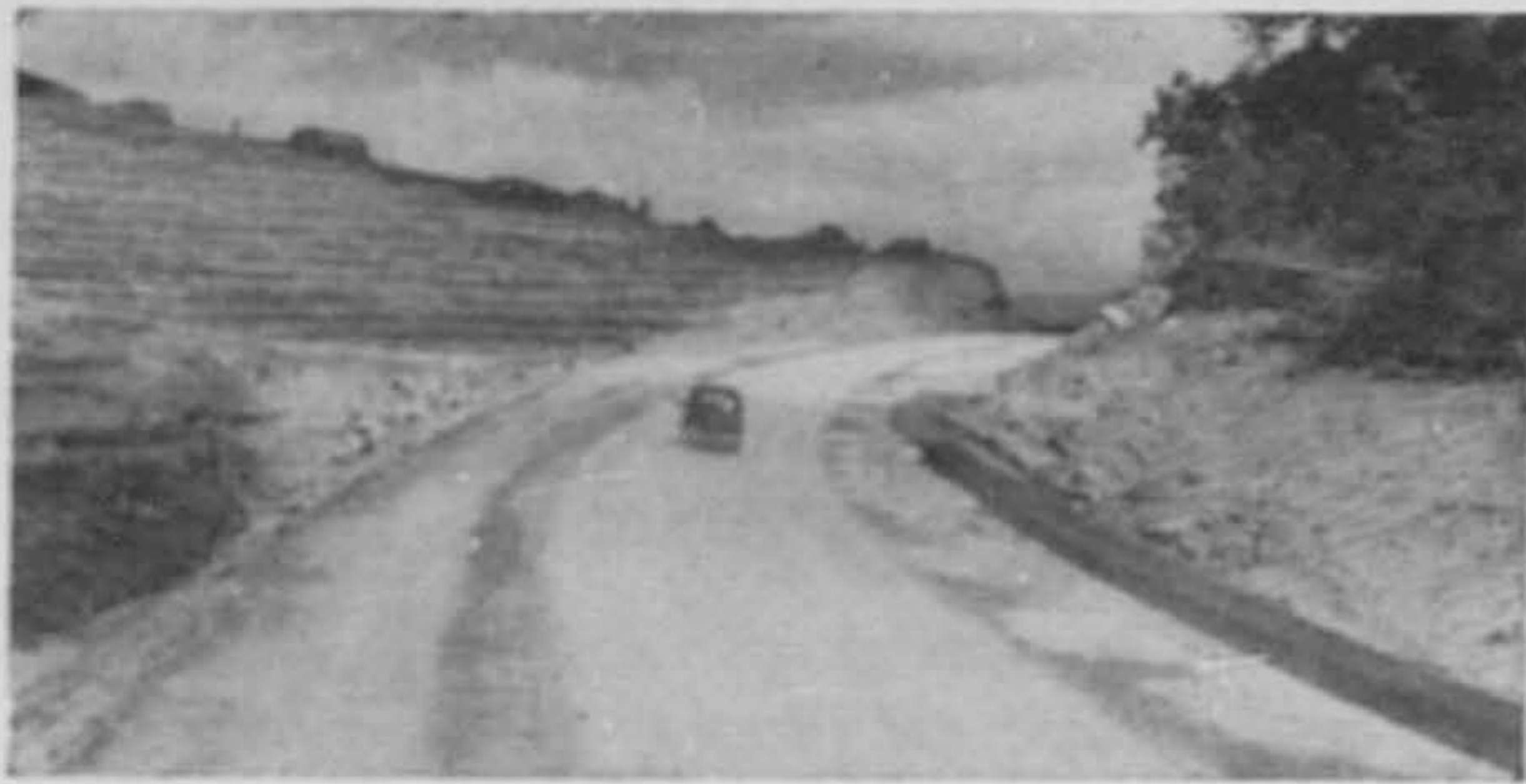
A broad laterite road serves as an approach road to Utan Percha Land Development Scheme in Malacca.
