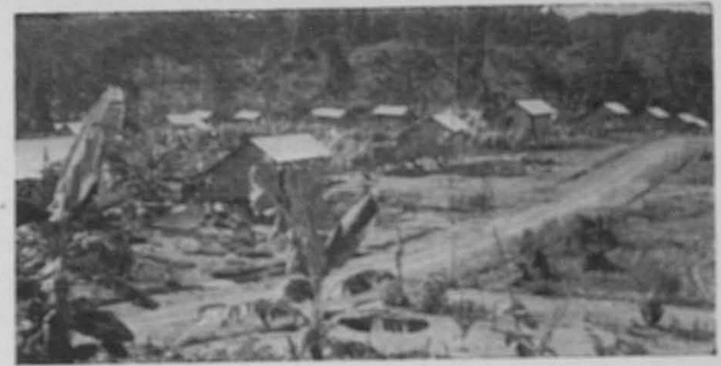
A general view of settlers low-cost housing in the Federal Land Development Scheme in Labu, Negri Sembilan.
