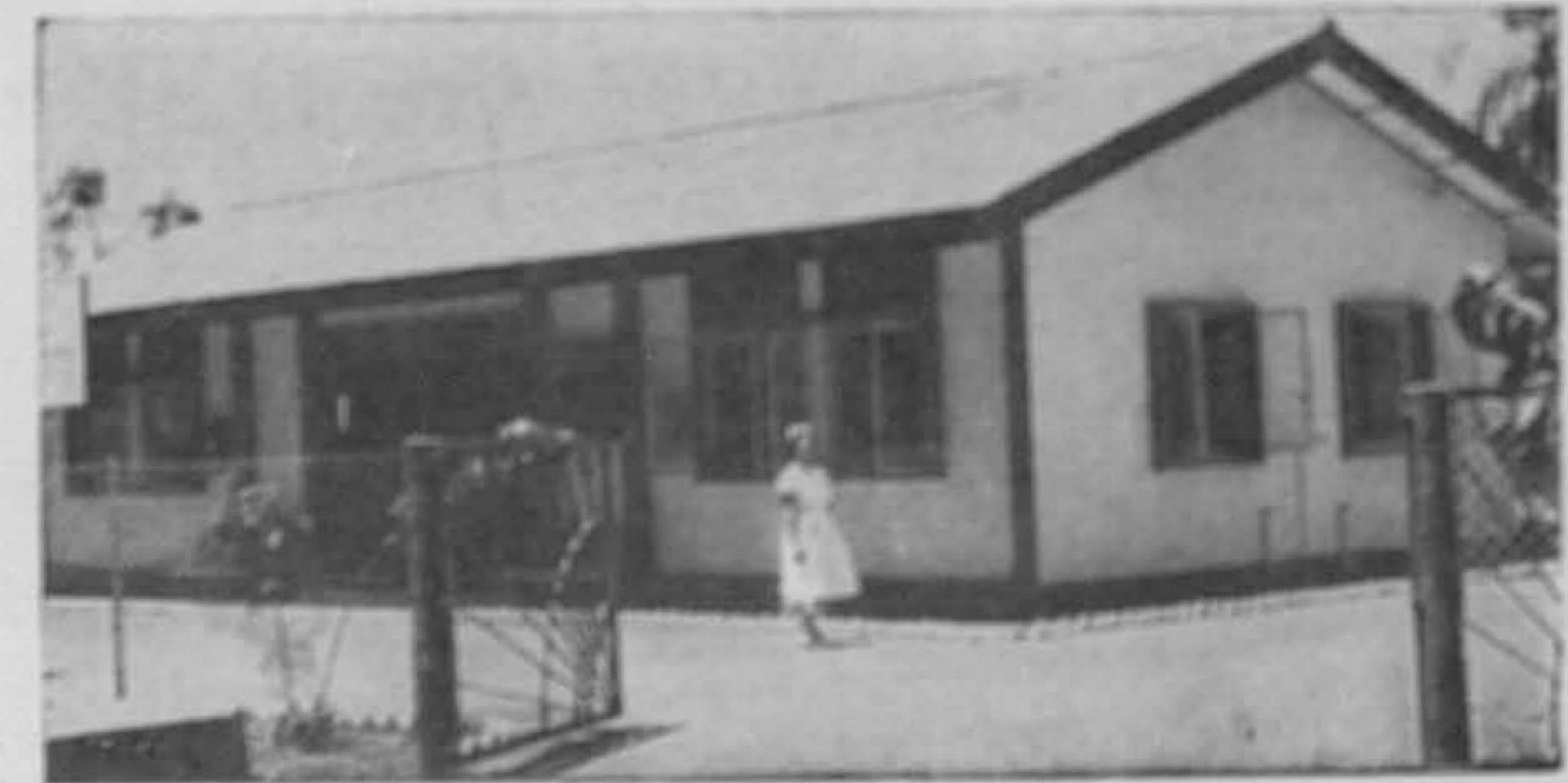
A new Sub-Health Centre in Perlis.
