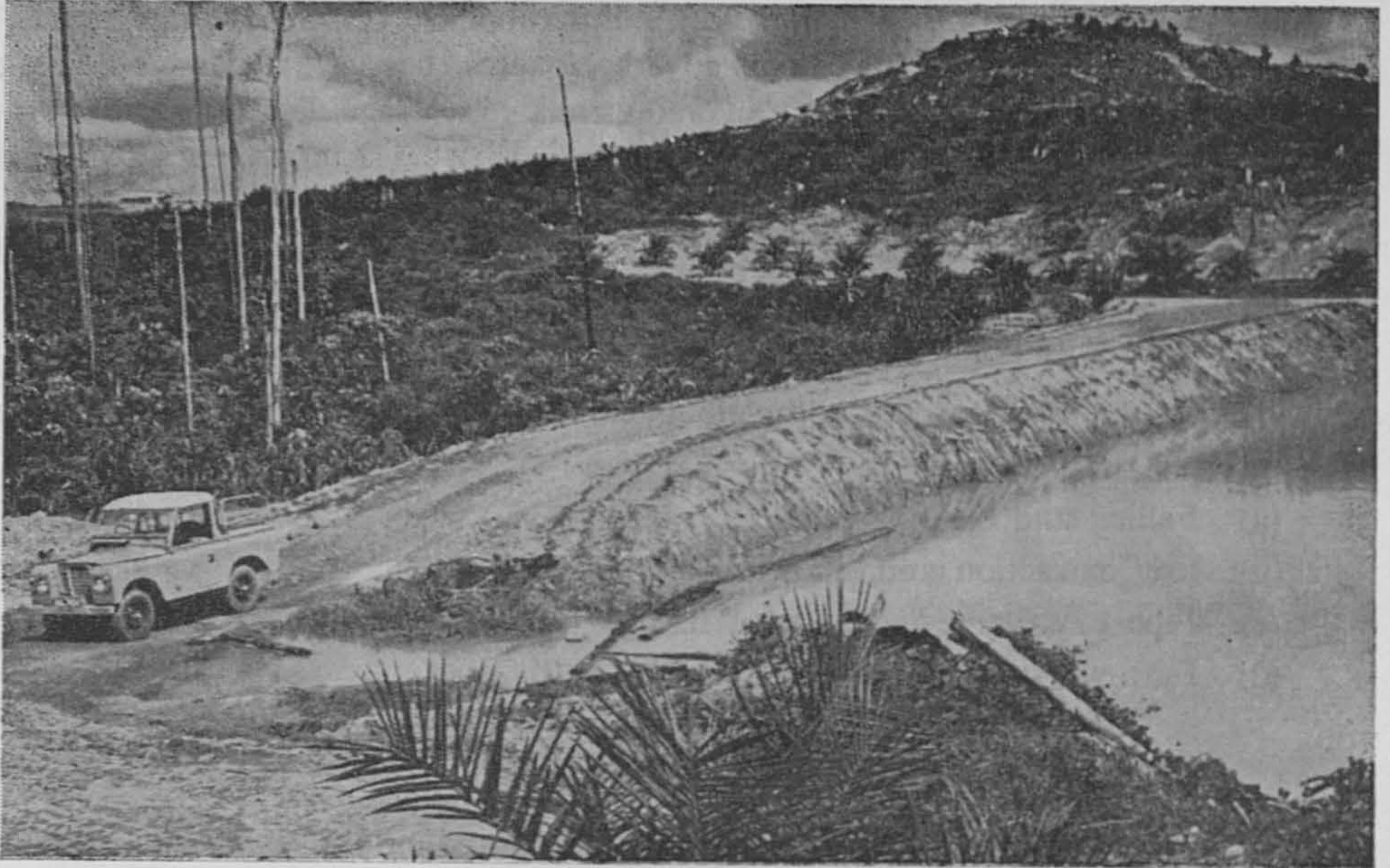
Figure 1. The dam at Kekayaan Estate with spillway at left of picture.
