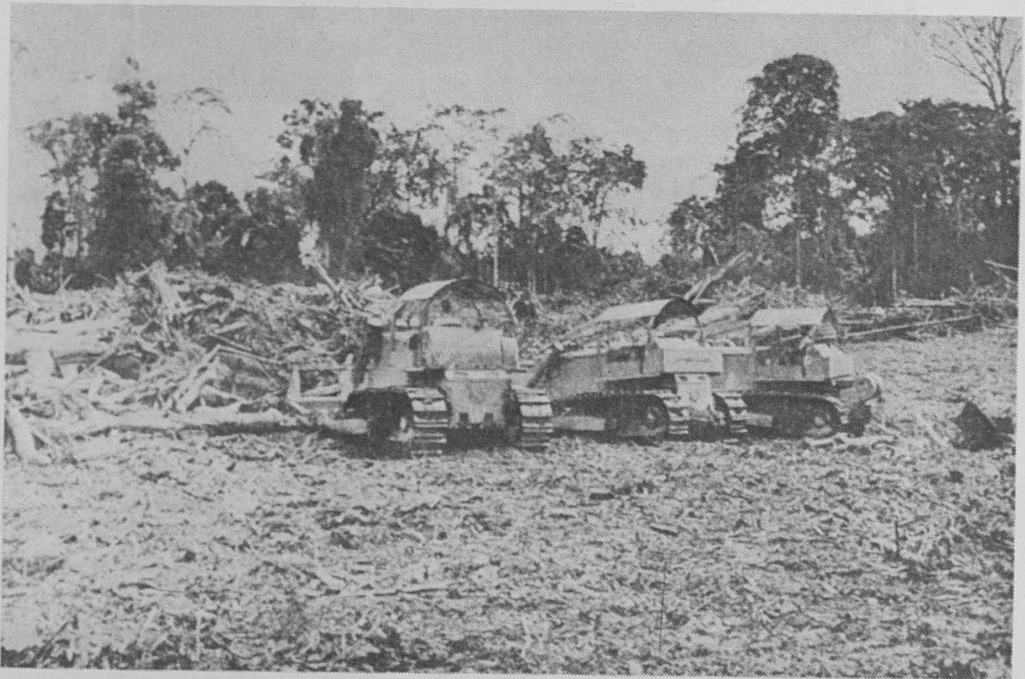
Figure 5. Squadron stacking using three tractors
