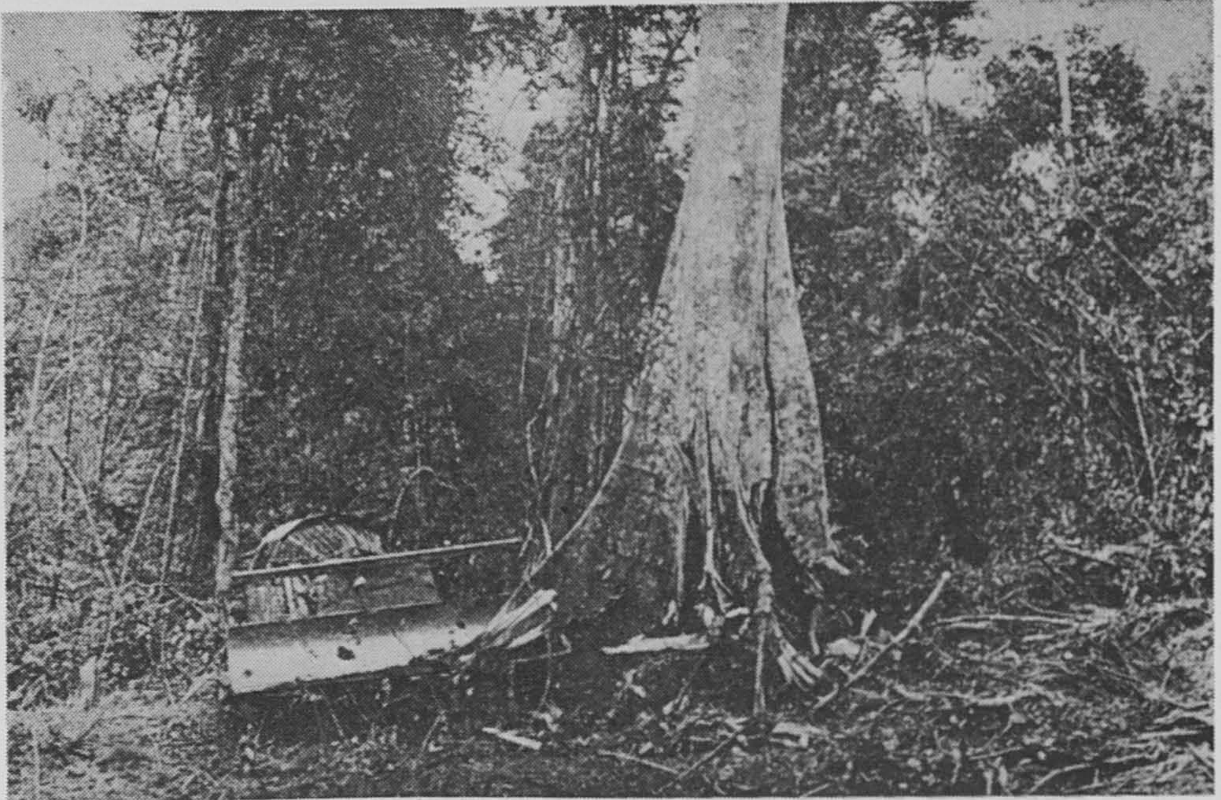
Figure 4. Felling with Rome KG blade
