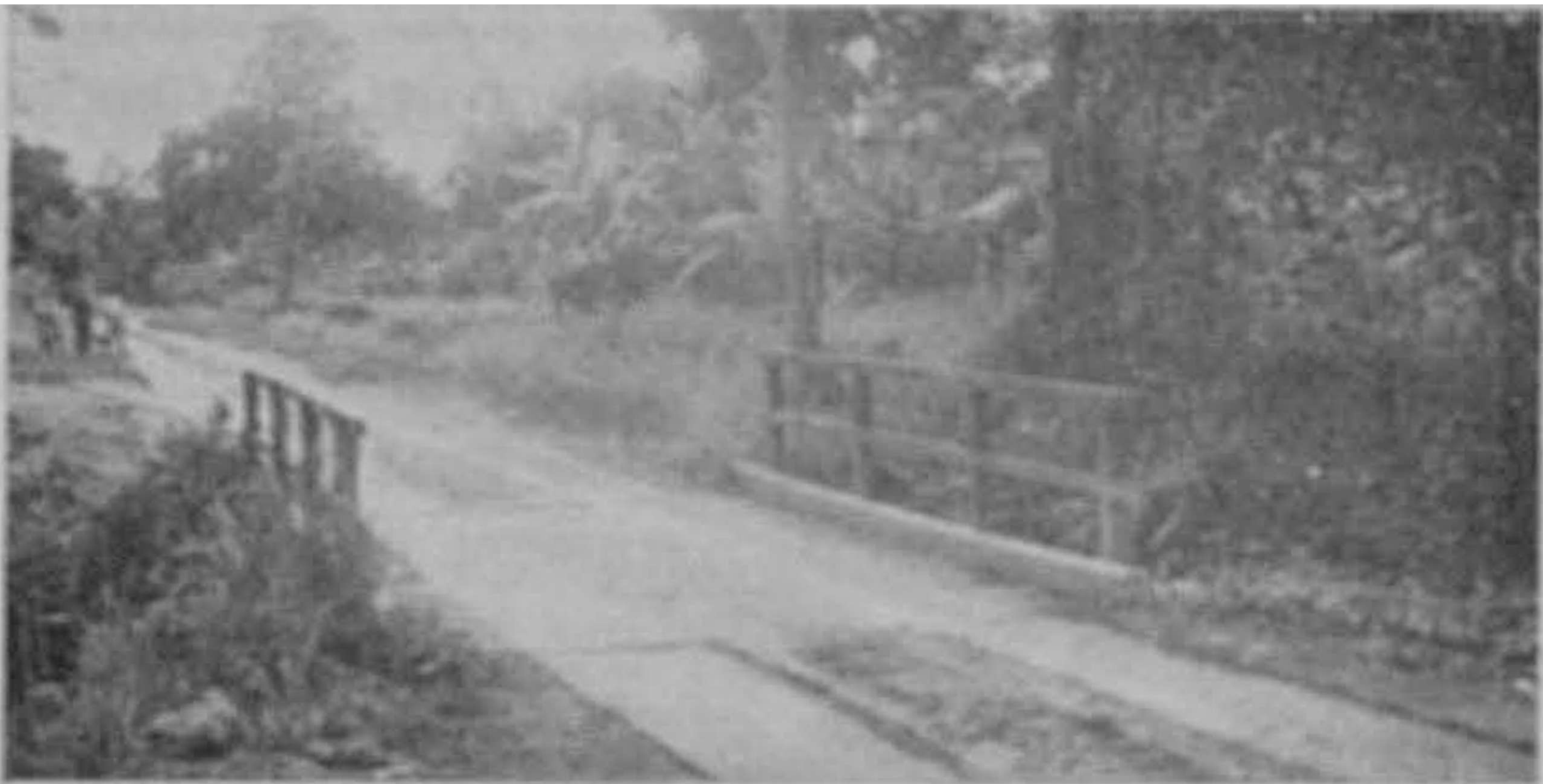
A kampong road with a new bridge provides access to secluded kampongs in the district of Gelang Patah in Johore.
