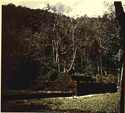
The Bukit Batu Pahat temple, Kedah: restored stone basement and plinth. See also Plate 9
