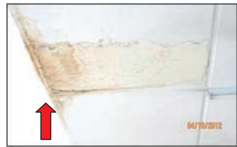
SK Nanga Ajau, Betong - Kesan Resapan Air Di Siling Asrama Lelaki A1 (04.10.2012)
