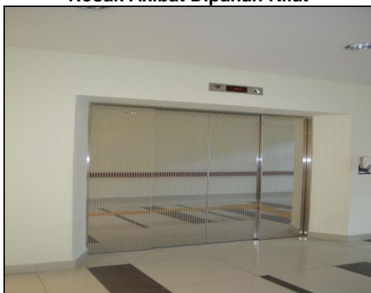
GAMBAR 6.19 Lif Di Medical Rehabilitation Block Yang Rosak Akibat Dipanah Kilat
