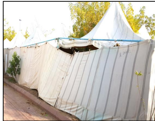
GAMBAR 9.11 Dinding Khemah Condong
