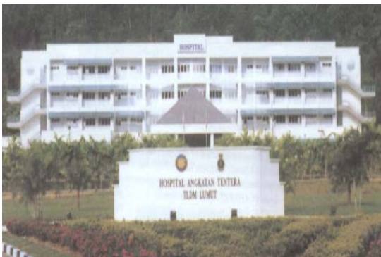
Hospital Lumut, Perak
