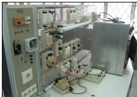
Politeknik Kuching - Electrical Installation Skills Trainer
