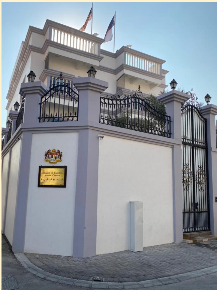
The new Chancery building of Embassy of Malaysia in Manama in Al Mahooz
