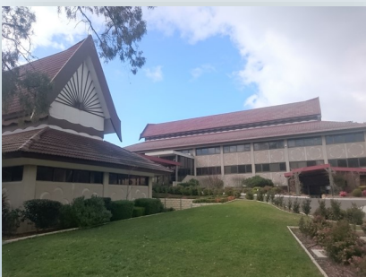
Current Chancery building at 7 Perth Avenue, Yarralumla
