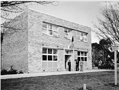
First Chancery building at Kingston, Canberra
