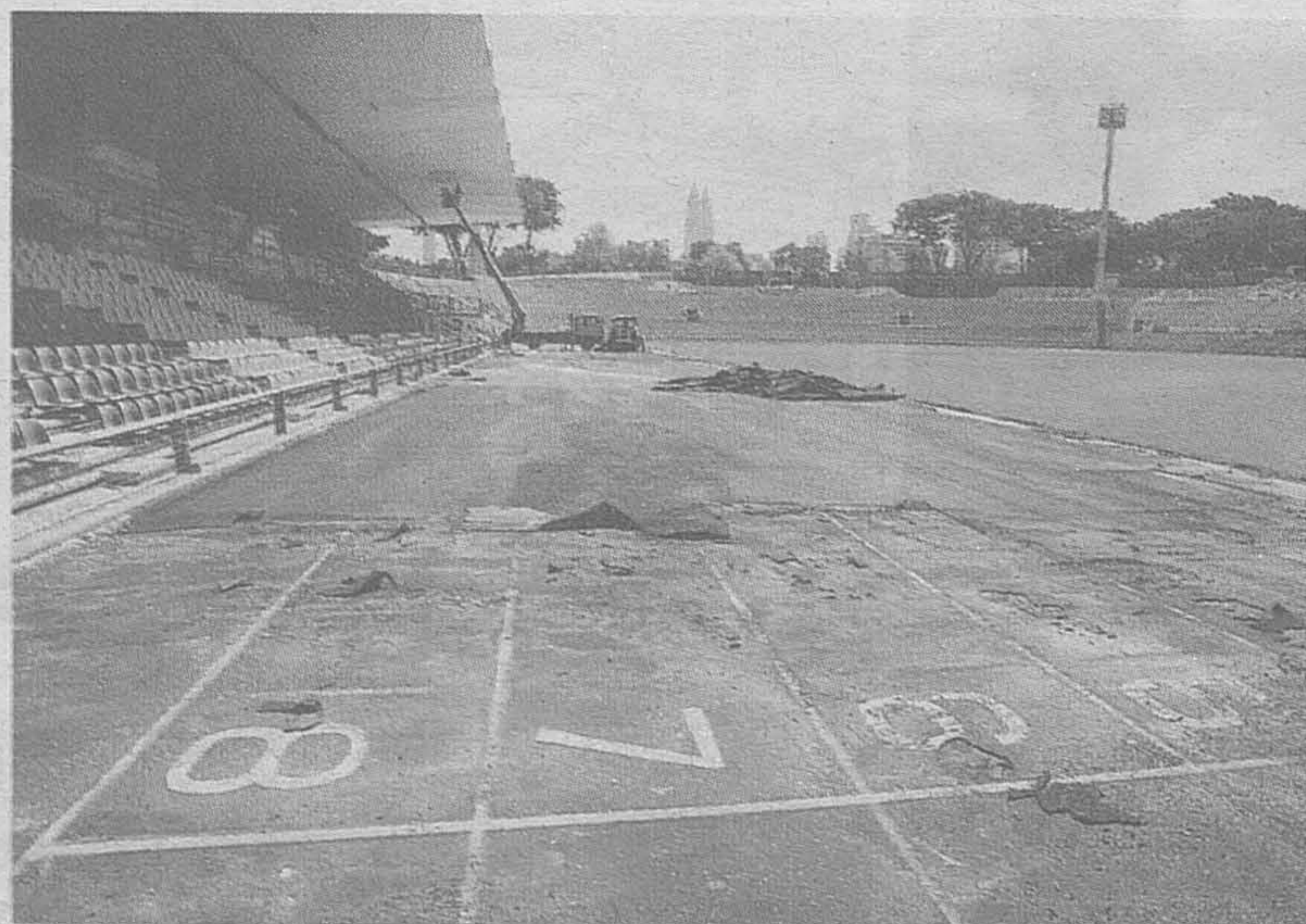
Removal: Workers are stripping the track laid for the 1989 SEA Games.
