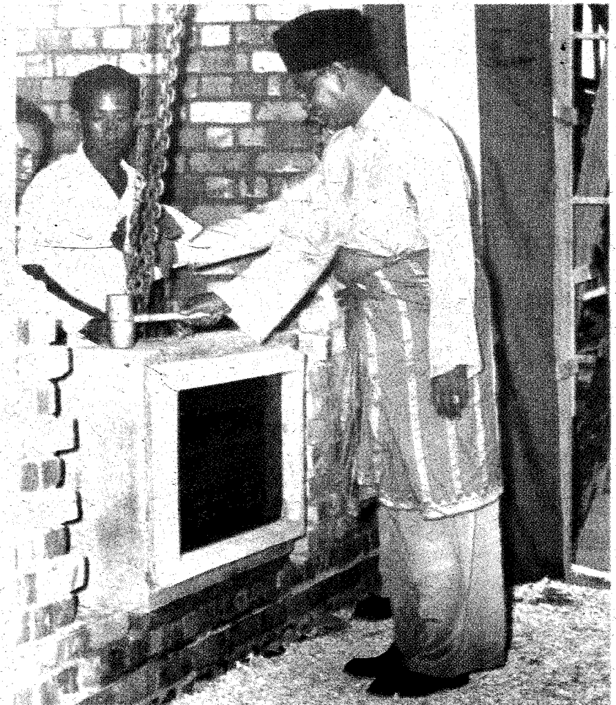
Tunku Abdul Rahman Putra Al-Haj laying the foundation stone of the Merdeka Stadium on Feb 15, 1957.
