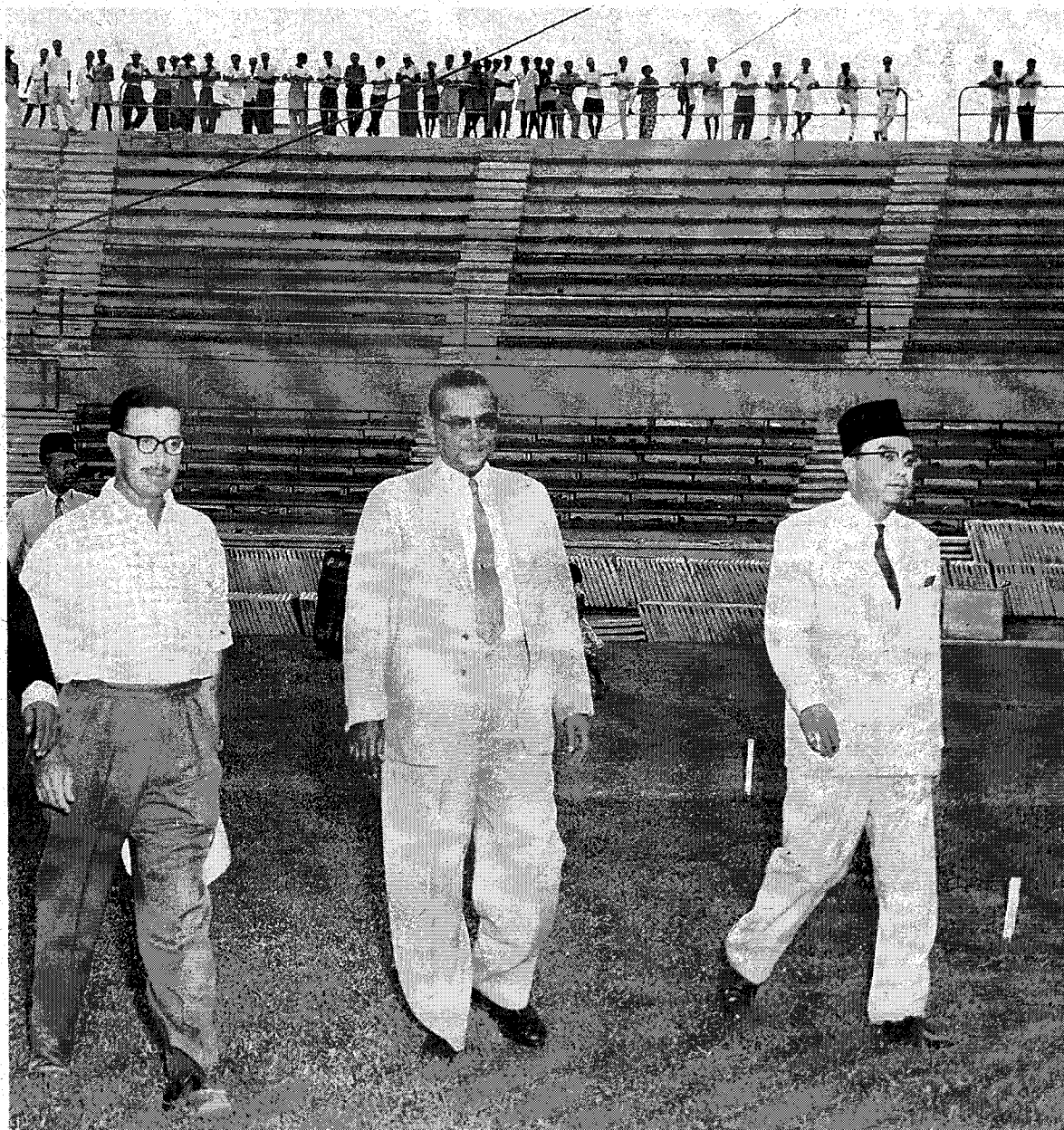
Tunku Abdul Rahman, flanked by Tun Abdul Razak and S.E. Jewkes, who was responsible for the planning, design and construction of Merdeka Stadium, visiting the worksite in June 1957. — File picture
