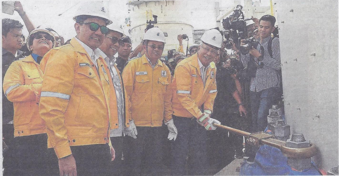
Najib using an adjustable spanner to tighten the screw of the fractionator to mark the completed installation of the tallest and heaviest process column in Malaysia
