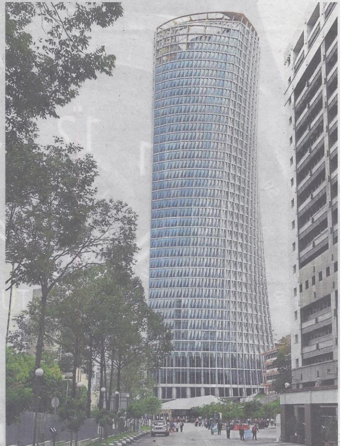
Standing tall and proud: Green building Menara Kerja Raya in full view.
