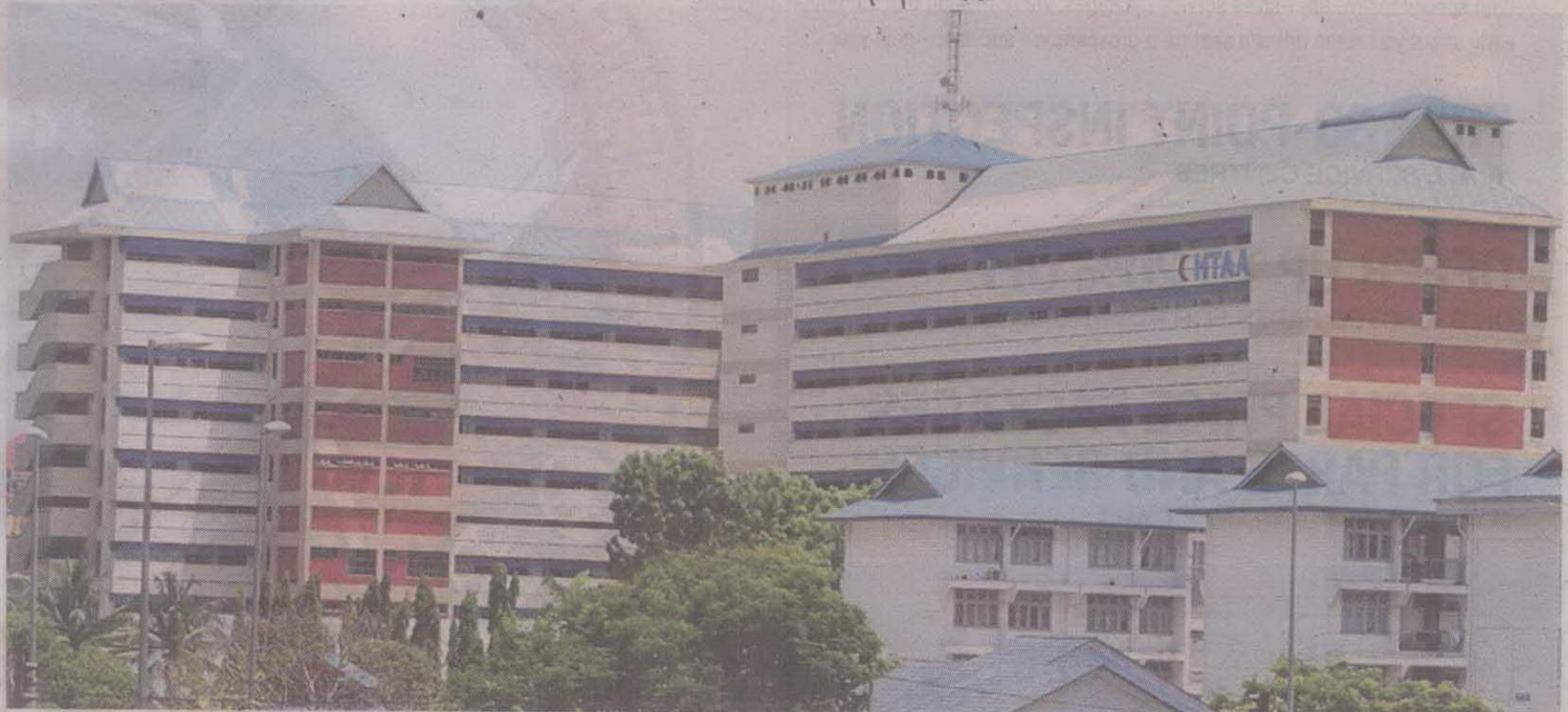
Repair works on the malfunctioning air-conditioning system at Hospital Tengku Ampuan Afzan , Kuantan, will reportedly take 18 months to complete .
