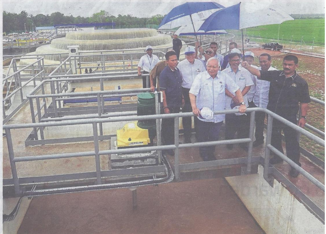
Site visit: Najib, accompanied by state officials, taking a look at the water filters during a ceremony to hand over the Ganchong water treatment plant to the Pahang government. — Bernama
