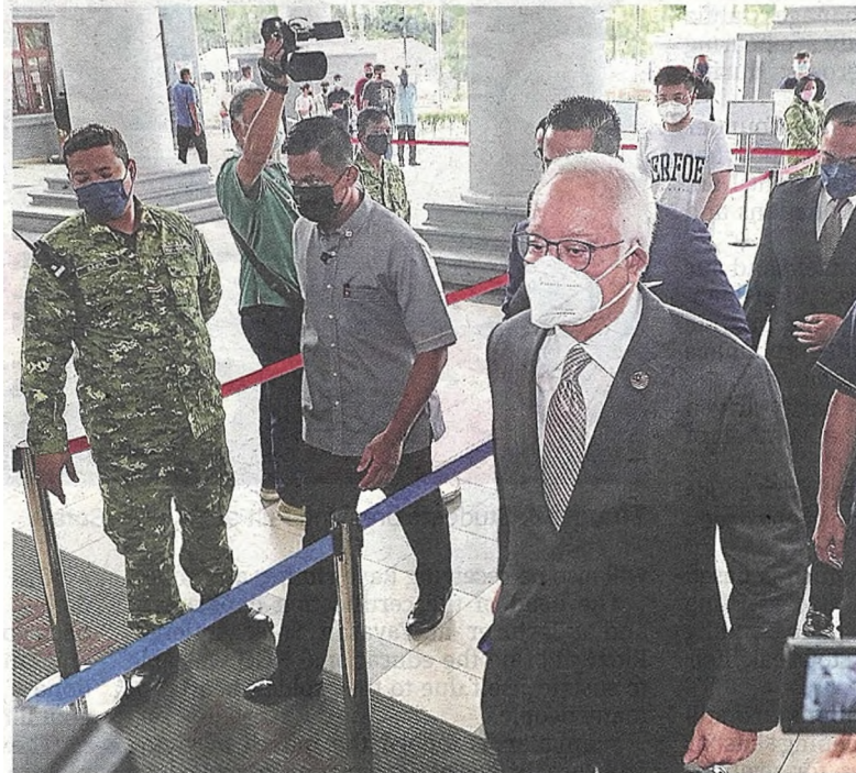
Ongoing case: Najib arriving at the Jalan Duta court complex in Kuala Lumpur for the 1MDB trial.
