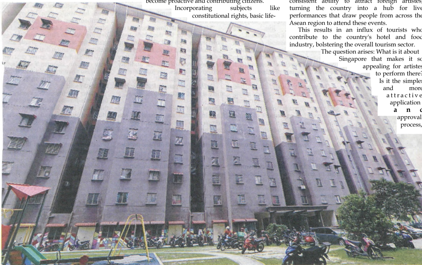
Many of the People's Housing areas have become unsuitable for living due to inadequate maintenance and poor waste management.
