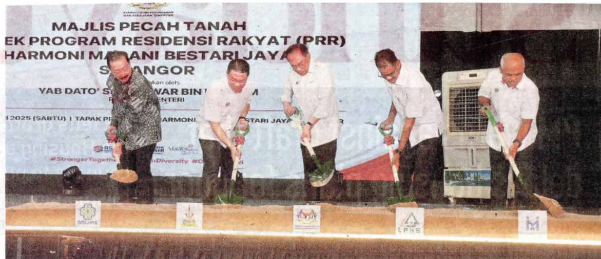
Prime Minister Datuk Seri Anwar Ibrahim (centre) shovelling soil during the groundbreaking for the Bestari Jaya People's Residency Programme in Kuala Selangor yesterday. With him are (from left) Berjaya Corporation Bhd founder Tan Sri Vincent Tan, Housing and Local Government Minister Nga Kor Ming, Selangor Human Resources and Poverty Eradication Committee chairman V. Papparaidu and Housing and Local Government Ministry secretary-general Datuk Noor Azman Talib. NSTP PIC BY FAIZ ANUAR
