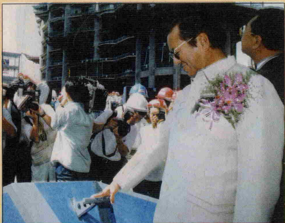
AND UP WE GO: Dr Mahathir pulling the lever to raise the Petronas Twin Towers skybridge's 325-tonne centre section to the 41st and 42nd floors of the tallest building in the world on Aug 7
