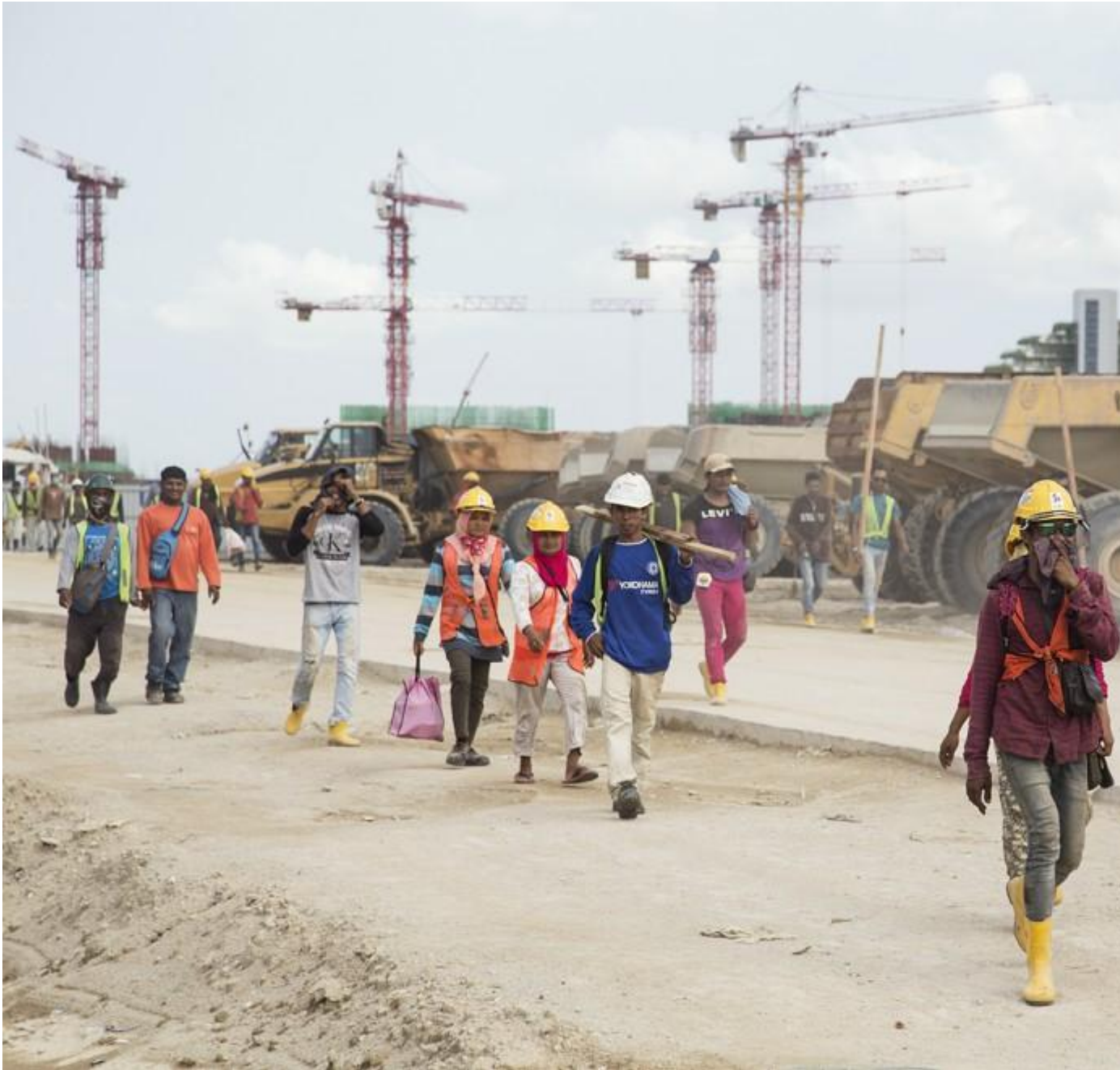
Workers at the construction site. Picture: Edward Hursta
