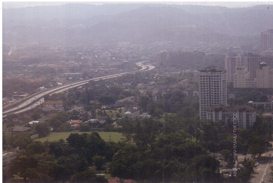
Highways traversing city and country are a lasting legacy of the Mahathir era. Pictured above is the Ampang elevated highway
