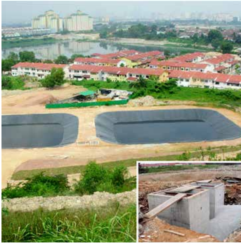
Leachate holding pond, part of the Taman Beringin Leachate Treatment Plant. (Inset) Leachate sump
