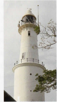
Kuala Selangor Lighthouse 85
