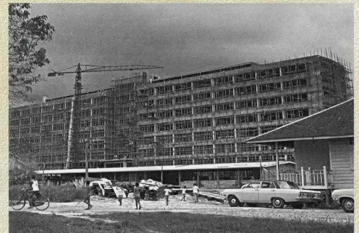
Sarawak General Hospital under construction - 1969.
