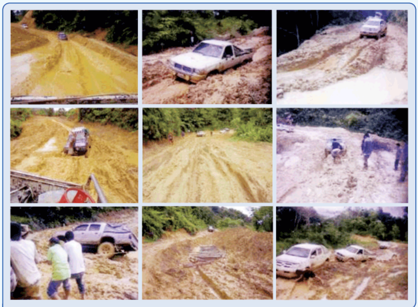
Figure 5: Poor conditions of logging roads needing remedial work
