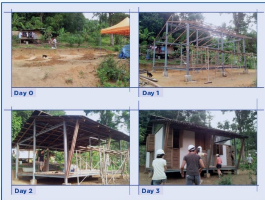
Figure 17: Modular housing construction process
