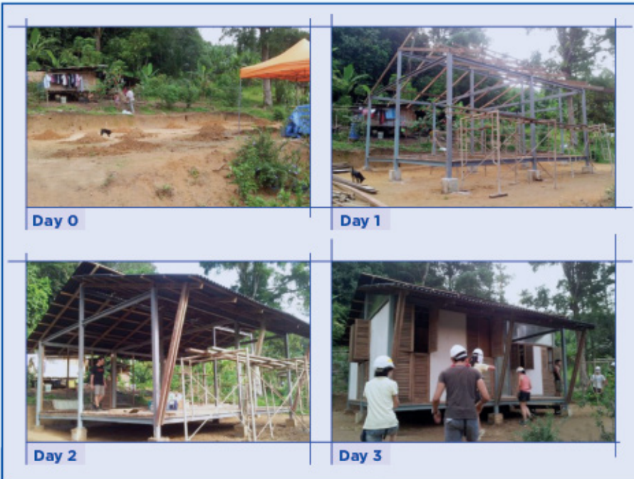
Figure 17: Modular housing construction process
